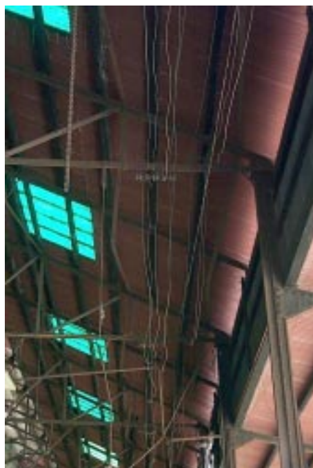
Left: Old electrical wiring suspended from the roof structure. Source: OC+P 2003
