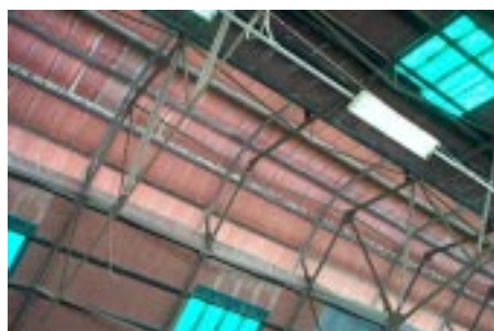
Bottom: View of roof showing counter trusses. Source: OC+P 2003
