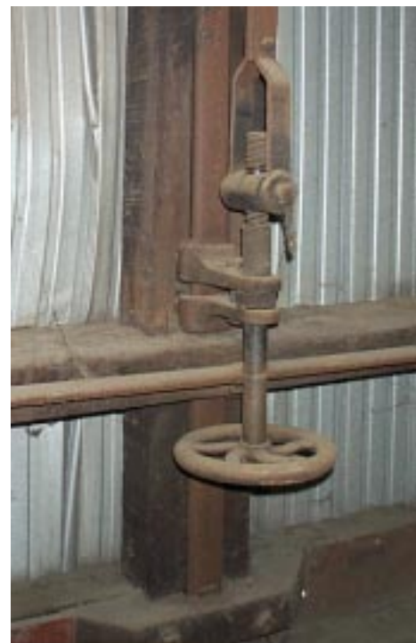
Opening mechanism for the louvres.
